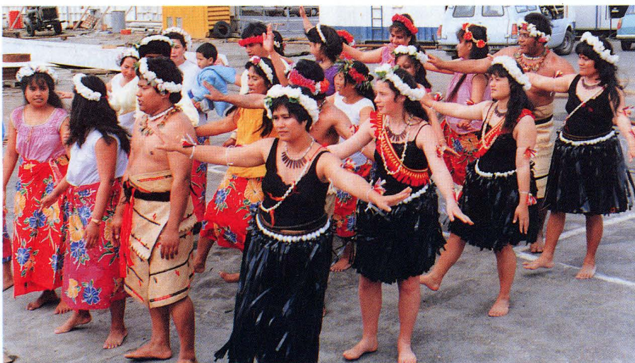
Members of Auckland's Kiribati community greet TARATAI with song and dance on the HOBSON WHARF building site.
